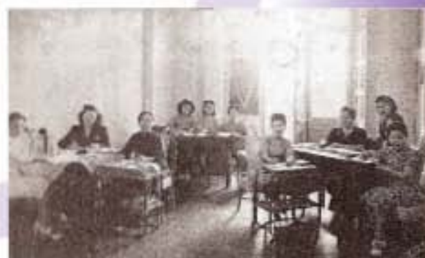
Resumption of work after the war
